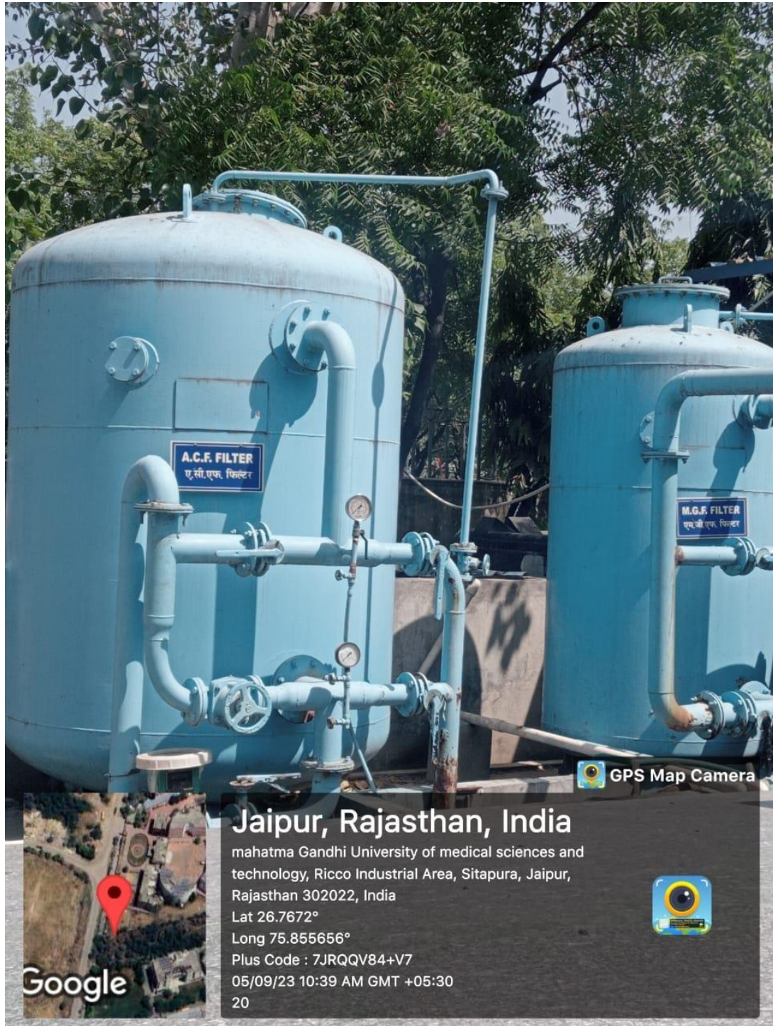
A.C.F. & M.G.F. FILTERS IN SEWAGE TREATMENT PLANT
